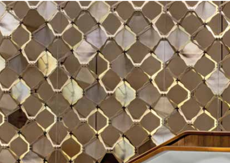
Screens made of powder-coated aluminium modules, enhanced with leather and textile. Project carried out for the cruise ship Celebrity Edge (Celebrity Cruises Inc). Partnership between Jouin Manku and Mathieu Bassée - mtb-paris.com
